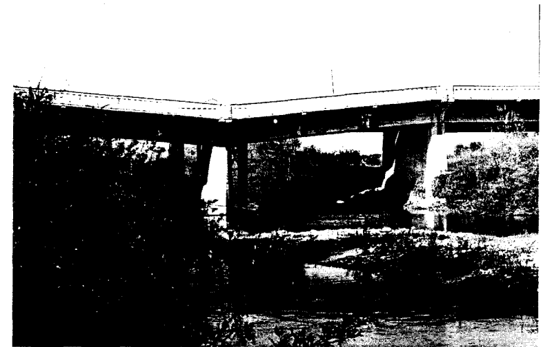
Figure 8.20 One of the mid-channel piers supporting this bridge sank about 1.5 m when it was undermined by scour in the river channel.
