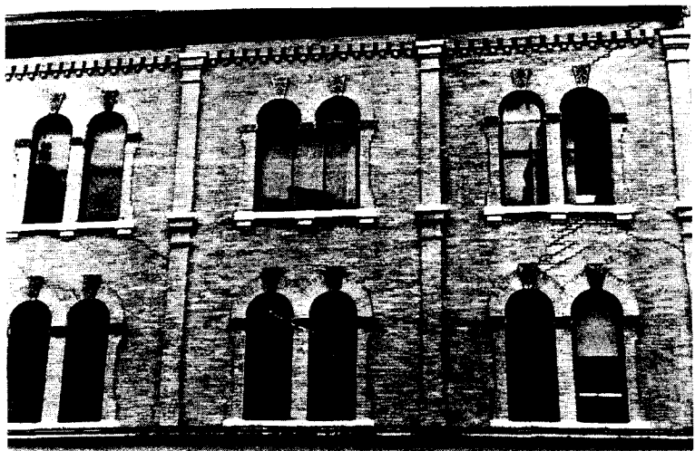
Figure 2.7 This old brick building has experienced excessive differential settlements, as evidenced by the diagonal cracks in the exterior wall.
