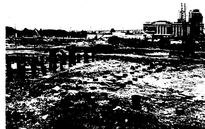
Figure 11.4 Groups of timber piles. Those in the foreground have been cut to the final head elevation (National Timber Piling Council).
