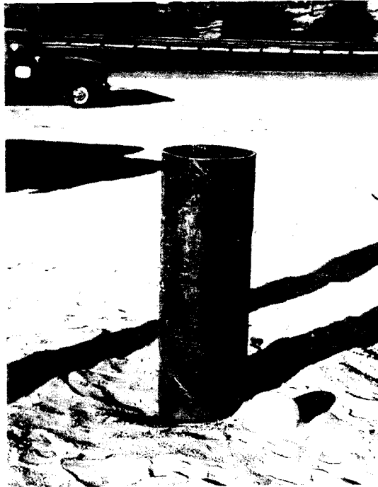
Figure 11.10 A 16 inch (406 mm) diameter steel pipe pile.
