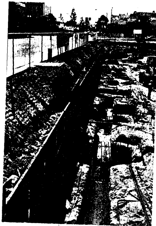
Figure 22.11 The ground surface at this site was originally level with the street. However, the proposed building, shown under construction, is to have a basement, so the site was excavated to a lower elevation. A soldier pile wall is being used to provide temporary support for the street. The permanent basement wall will be located directly above the grade beam shown in the foreground, and the columns above the pile caps will be embedded in the exterior wall. Once this permanent wall is in place, the zone between it and the street will be backfilled and the timber lagging will be removed. The steel sheet piles may or may not be removed.
