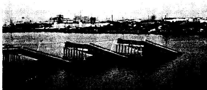
Figure 17.4 The Showa Bridge in Niigata, Japan, collapsed due to the formation of lateral spreads in the underling soils during the 1964 earthquake. These lateral spreads pushed the pile foundations out of position, thus removing support from the simply-supported deck (Earthquake Engineering Research Center Library, University of California, Berkeley, Steinbrugge Collection).
