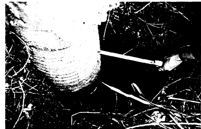
Figure 17.5 This pile, which supported a bridge near Watsonville, California, moved laterally during the 1989 Loma Prieta Earthquake, creating a gap between the pile and the soil. The size of this gap is an indication of the excessive lateral deflections that occurred during the earthquake (Loma Prieta Collection, Earthquake Engineering Research Center, University of California, Berkeley).
