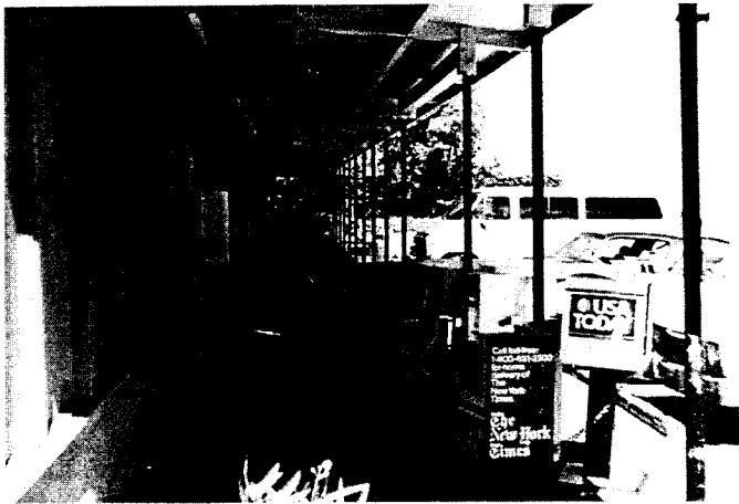
Figure 18.4 The ground around this pile-supported supermarket building settled about 400 mm in twenty-five years, but the building remained at essentially the same elevation. This required continual maintenance around the perimeter of the building. Note the steep slope to reach the front door and the spacer blocks required at the top of the footing-supported posts (which settled with the surrounding ground).
