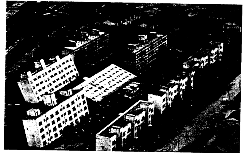
Figure 8.9 The soils beneath these apartment buildings in Niigata, Japan liquified during the 1964 earthquake, which produced bearing capacity failures. These failures reportedly occurred very slowly, and the buildings were very strong and rigid, so they remained virtually intact as they tilted. Afterwards, the occupants of the center building were able to evacuate by walking down the exterior wall (Earthquake Engineering Research Center Library, University of California, Berkeley, Steinbrugge Collection).
