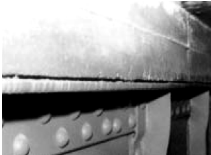
Figure 4.9 Crevice corrosion between concrete and steel
