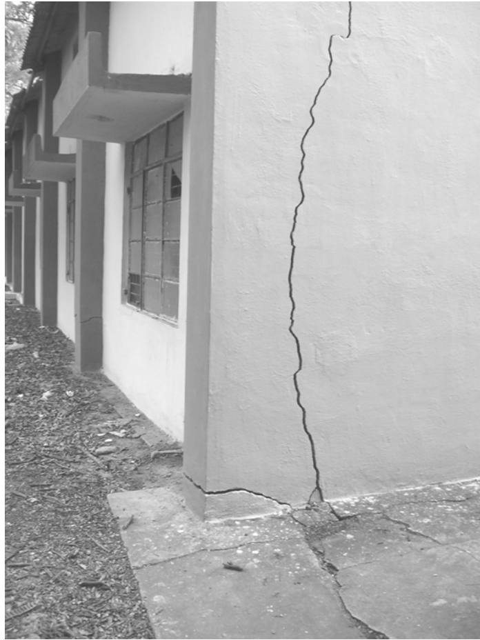
Figure 6.2b Vertical crack
