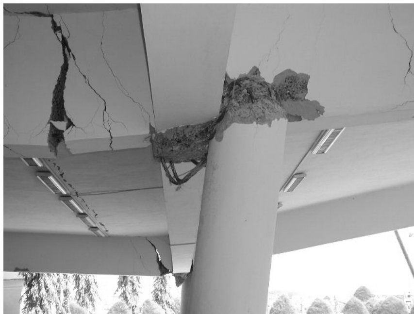
Figure 0.43 Failures in beam and column (Andaman earthquake, 2004)
