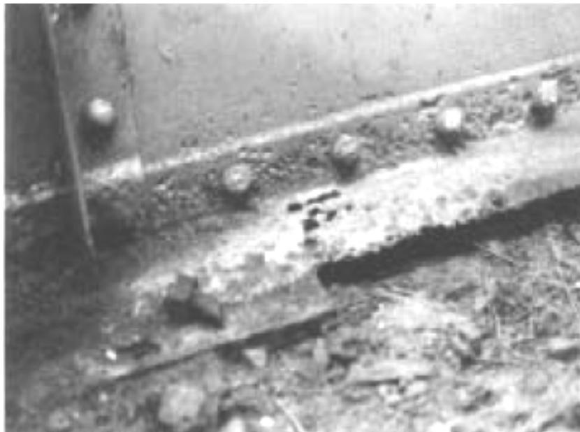
Figure 4. 7 Pitting corrosion of steel
