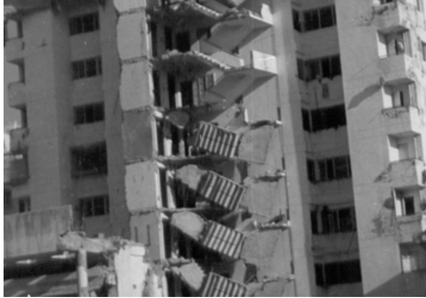
Figure 0.25 Collapse of overhanging projections (Bhuj earthquake, 2001) (Ref: www.nicee.org )
