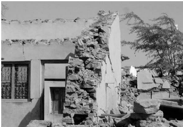
Figure 0.12 Collapse of brittle and poorly bonded stone masonry walls (Latur earthquake, 1993) (Ref: www.nicee.org )
