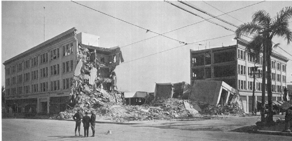
Figure 0.19 Collapse of an “L” shaped building (Macedonia earthquake, 1963)
