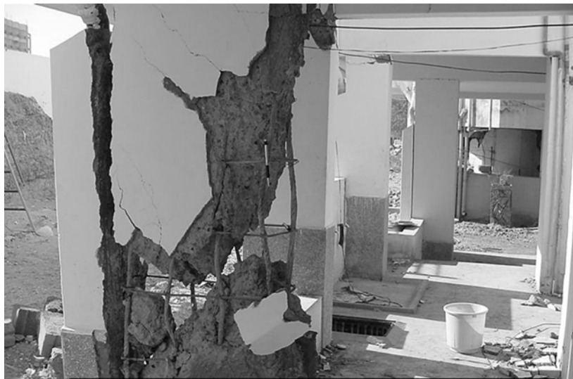
Figure 0.41 Shear failure in a reinforced concrete column (Ref: www.nicee.org )
