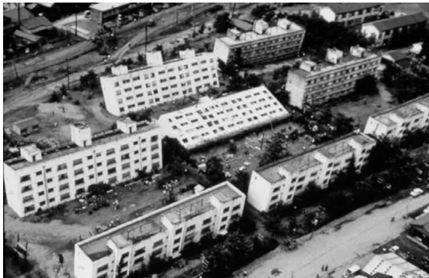
Figure 0.28 Buildings tilted due to liquefaction of soil (Niigata earthquake, Japan, 1964)
