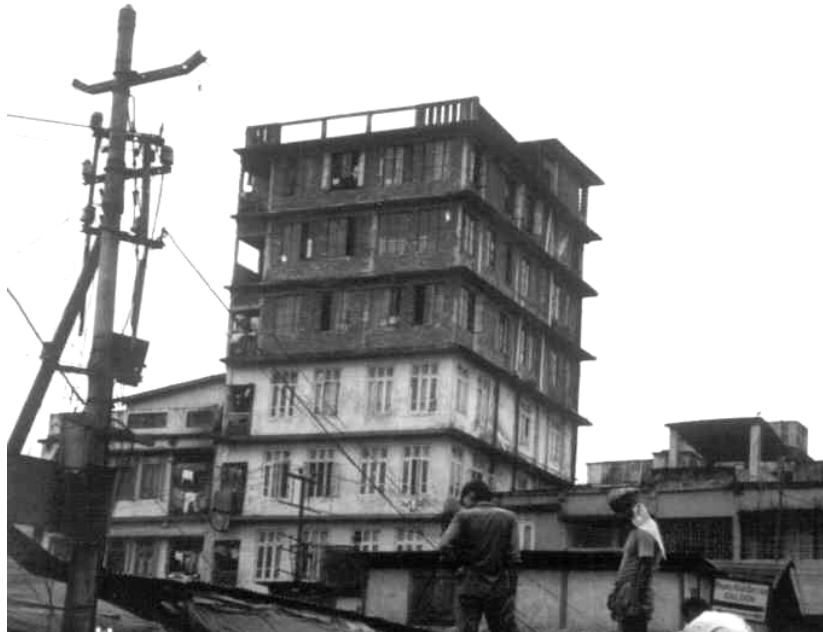
Figure 0.8 A 4-storeyed old building (in zone V) extended to 7-storey!
