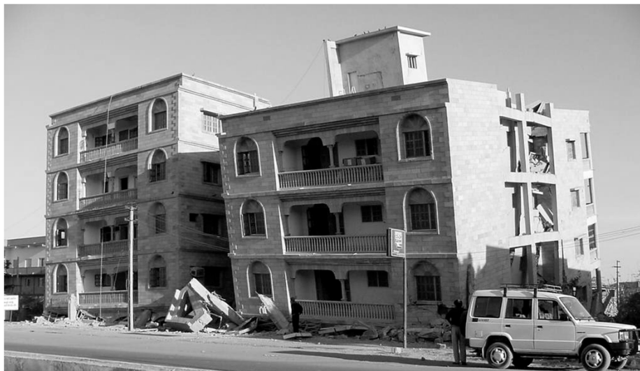
Figure 0.15 Collapse of the ground storey of a building (Bhuj earthquake, 2001) (Ref: www.nicee.org )
