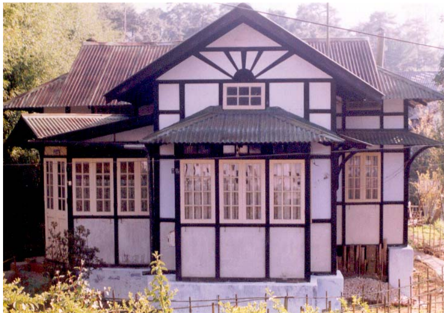
Figure 0.7 “Assam type” low-rise and light building
