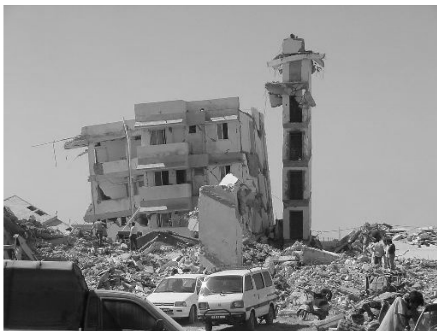
Figure 0.45 Lack of integrity between lift core and rest of the building (Bhuj earthquake, 2001) (Ref: www.nicee.org )
