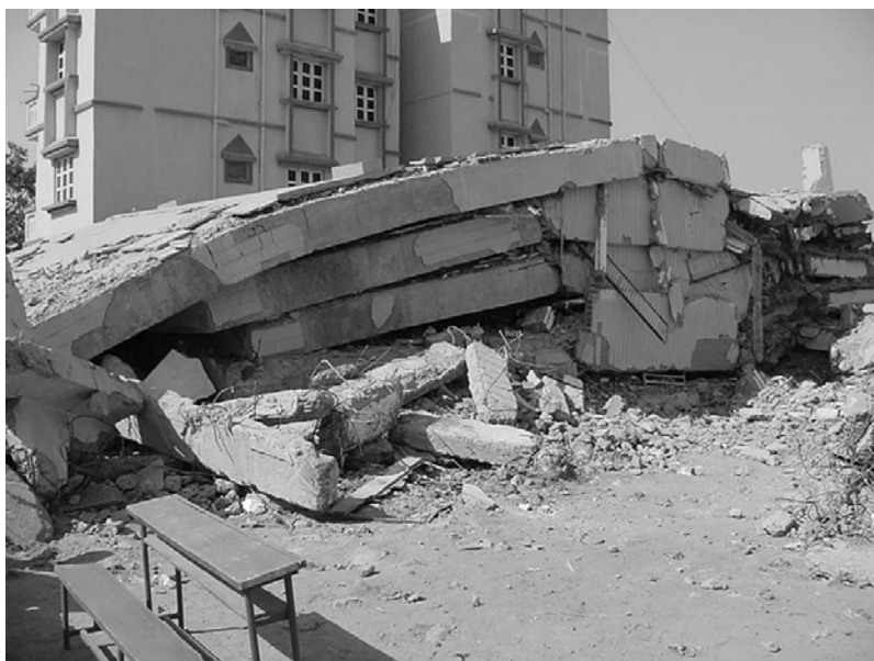
Figure 0.44 'Pancaking' failure due to failure in columns (Bhuj earthquake, 2001) (Ref: www.nicee.org )
