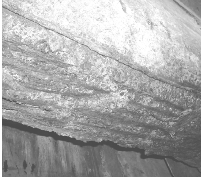
Figure 4.5 Severe corrosion damage to underside of a beam
