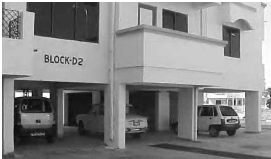
Figure 0.22 Building with open ground storey (Ref: www.nicee.org )
