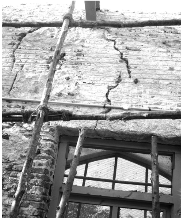
Figure 4.2 Vertical cracks in a brick masonry building
