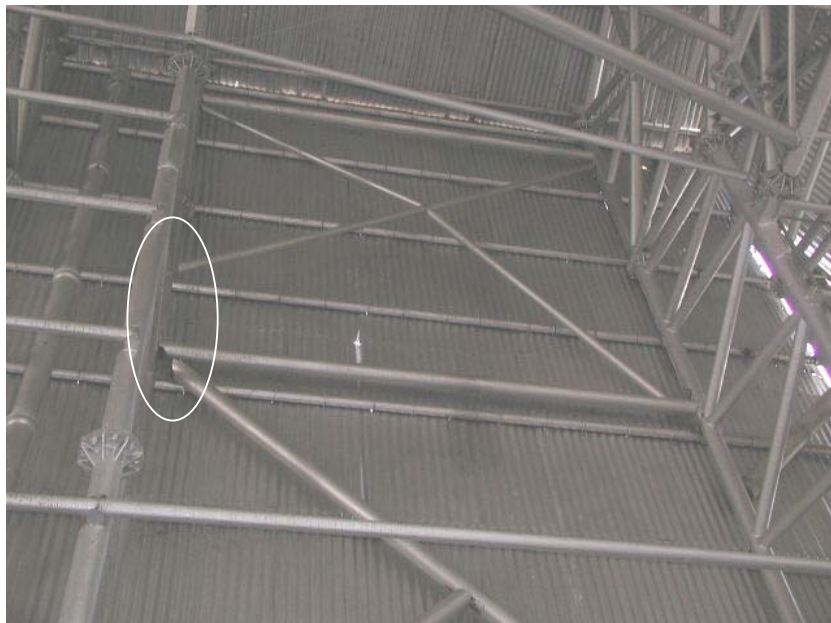
Figure 10.8 Failure of the end connections of braces (circled)
