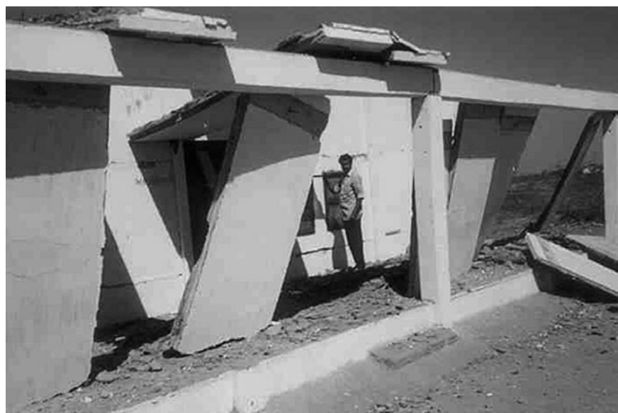
Figure 0.49 Lack of integrity in pre-cast construction (Bhuj earthquake, 2001) (Ref: www.nicee.org )
