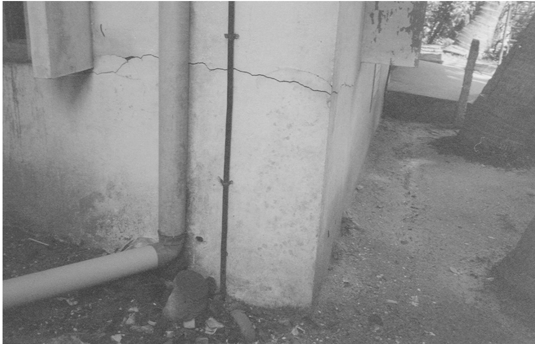
Figure 6.2a Horizontal crack
