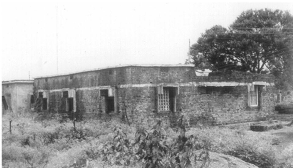
Figure 0.17 A masonry building with lintel band after 1993 Killari Earthquake: good integral action (Ref: www.nicee.org )
