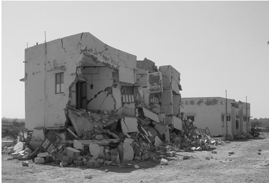
Figure 0.35 Lack of integrity due to absence of bands (Ref: www.nicee.org )
