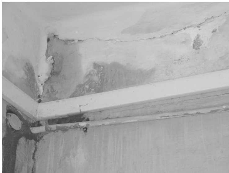
Figure 4.4 Cracking in a beam from corrosion of steel due to water seepage
