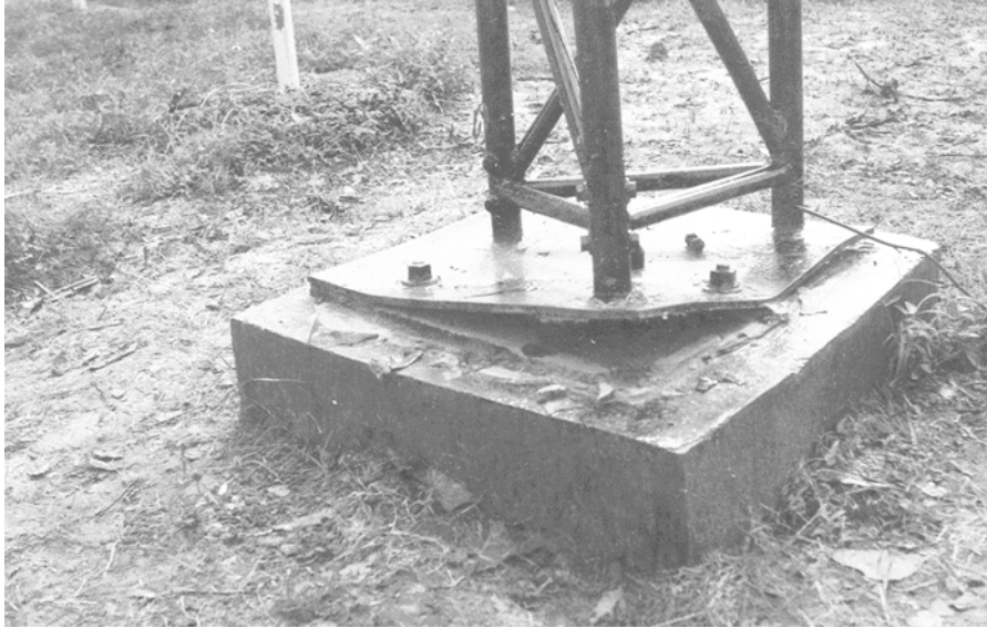
Figure 12.10 Damage in a base plate
