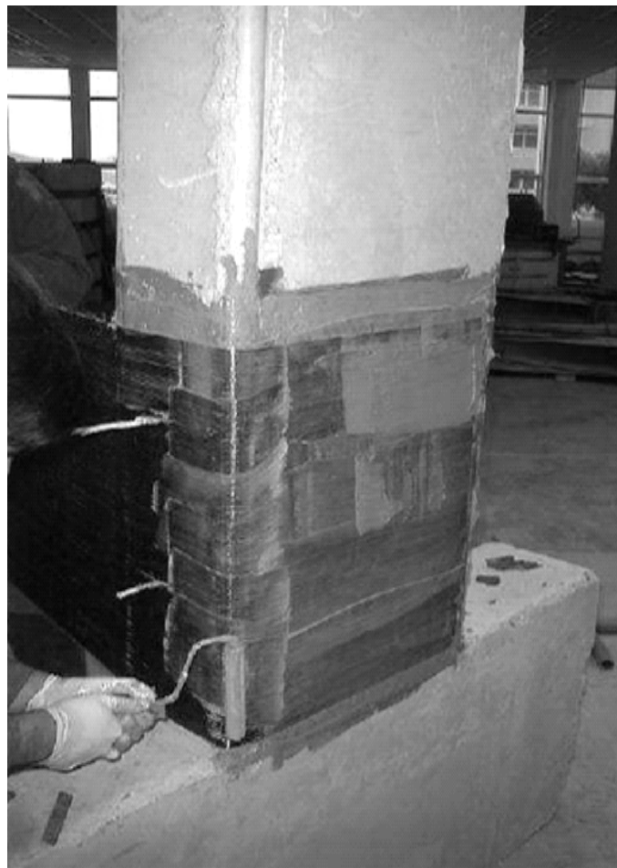
Figure 13.10 Wrapping of column using FRP composites
