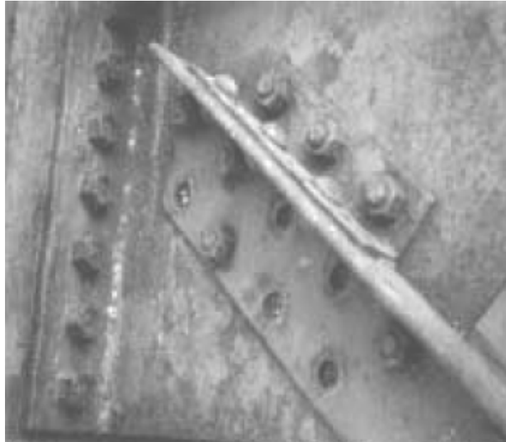
Figure 4. 8 Stress corrosion of bolts
