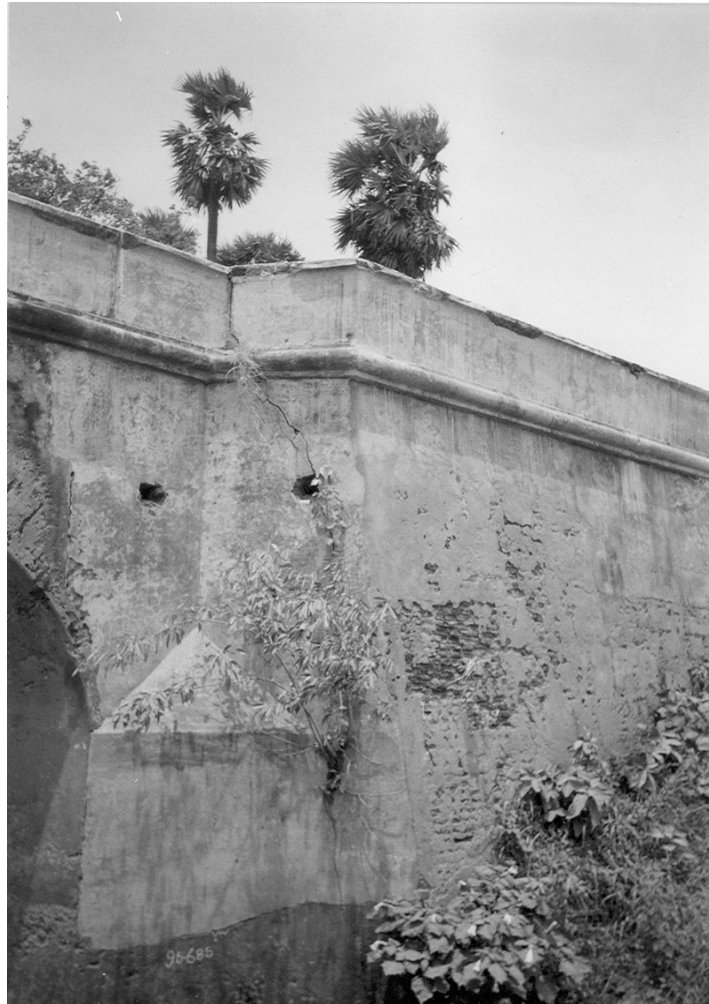
Figure 6.3 Deterioration of brick masonry due to spalling
