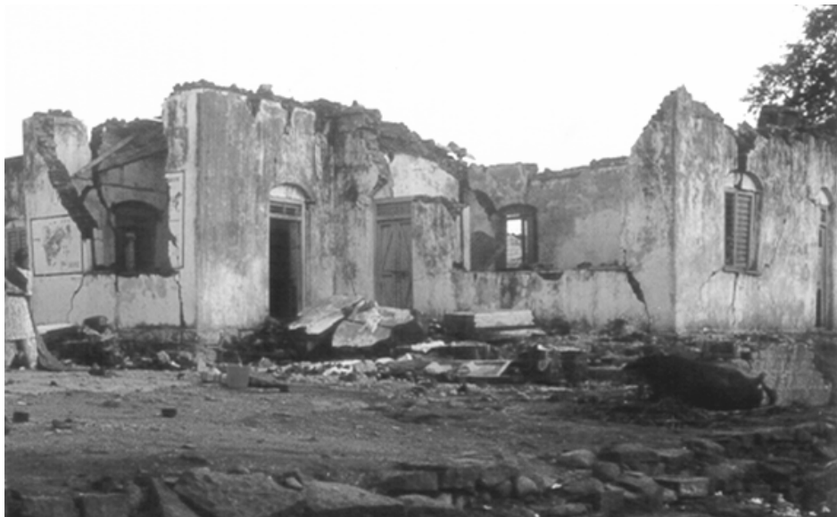
Figure 0.16 Poor integrity in a masonry building (Latur earthquake, 1993) (Ref: www.nicee.org )
