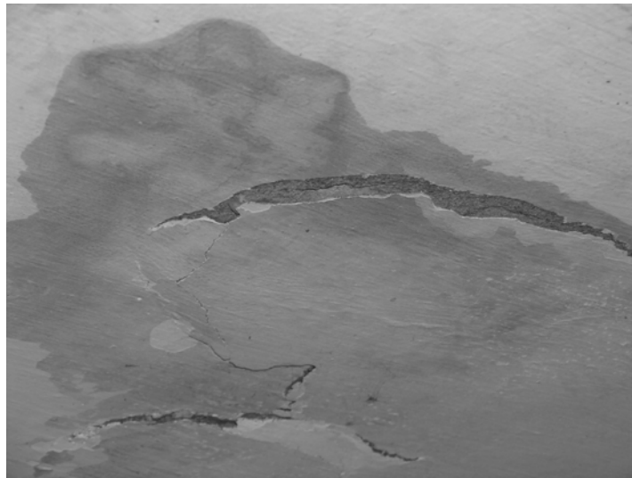
Figure 4.6 Delamination in a slab from corrosion of steel due to water seepage
