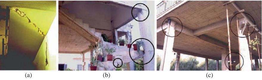
Plate 4 (a) Stair flight failing in shear as an inclined wall element in its strong direction; (b) corner stair in an open ground floor causes damage to the column it is connected to at mid-storey; and (c) columns at the diagonally opposite corner of the building failed during torsional response due to the stair in (b) – shown near bottom right at the back. (See also Figure 2.13 on page 82)
