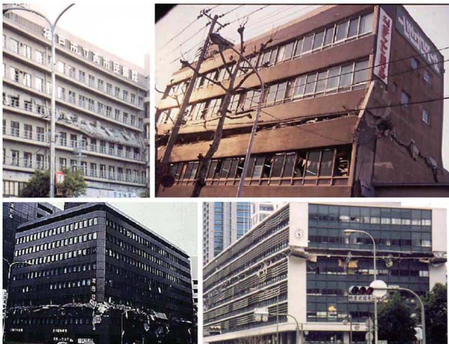
Fig. 2.4 Middle-storey collapses due to abrupt changes in stiffness or resistance of vertical elements (Kobe 1995)
