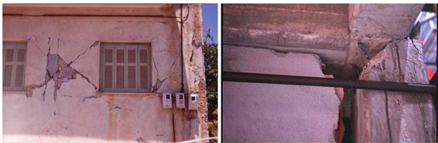
Fig. 2.11 Examples of shear failure of weak columns interacting with strong infills. (See also Colour Plate 2 on page 771)
