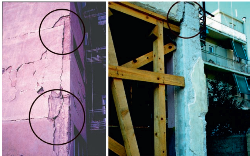
Plate 8 Pull-out of beam bars from short anchorage in corner joint has produced fixed-end rotation during the response and wide residual cracks (See also Figure 3.29 on page 208)
