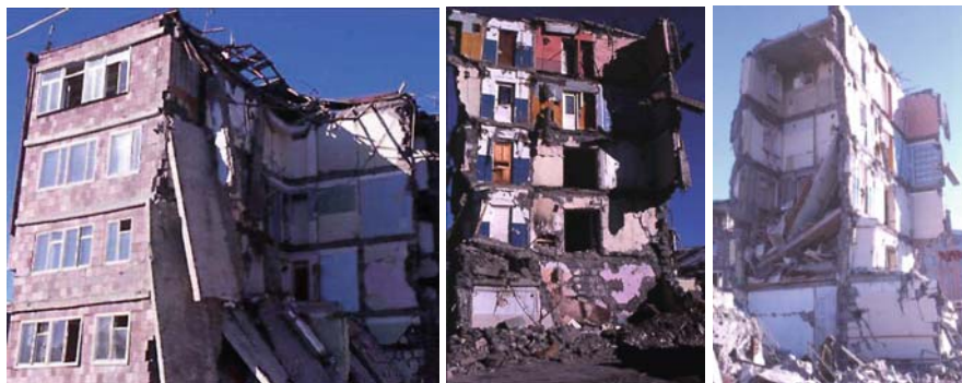
Fig. 2.6 Collapse of buildings with precast floors inadequately connected to the walls (Spitak, Armenia, 1988)
