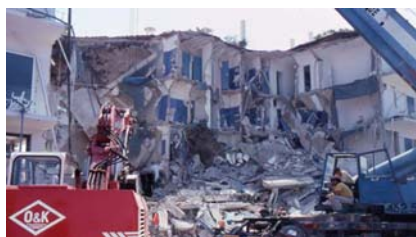
Fig. 2.24 Collapsed hotel in Aegio (GR): (a) framing plan of standard floor; (b) façade frame intact; (c) collapsed part with the frame surrounding the staircase shown at the far-right
