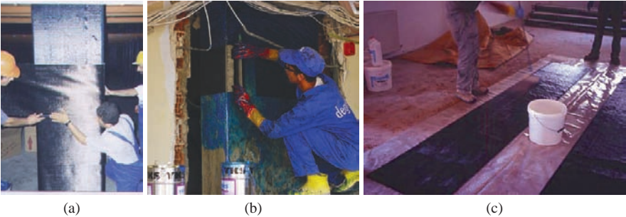
Plate 15 Hand lay-up of FRPs in situ: (a), (b) dry fabric impregnated in place (courtesy A. Ilki); (c) impregnation of the fabric right before placing (See also Figure 6.3 on page 654)
