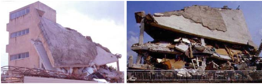
Fig. 2.1 Collapse of a building due to torsional response about a stiff shaft at the corner, Athens (1999) earthquake
