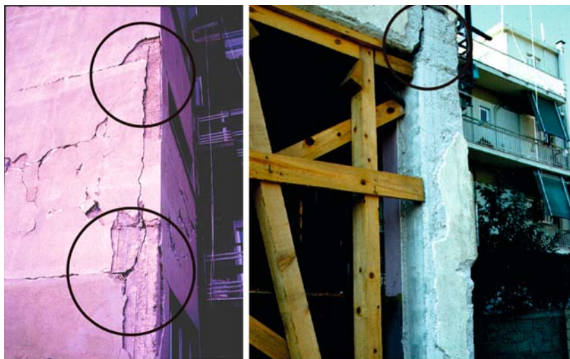
Fig. 3.29 Pull-out of beam bars from short anchorage in corner joint has produced fixed-end rotation during the response and wide residual cracks (See also Colour Plate 8 on page 722)
