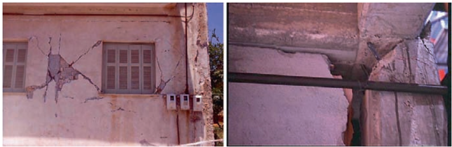
Plate 2 Examples of shear failure of weak columns interacting with strong infills. (See also Figure 2.11 on page 79)
