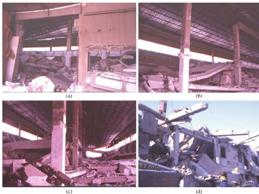
Fig. 2.7 Collapse of precast concrete buildings: (a)–(c) in Athens 1999; (d) in Spitak (Armenia) 1988
