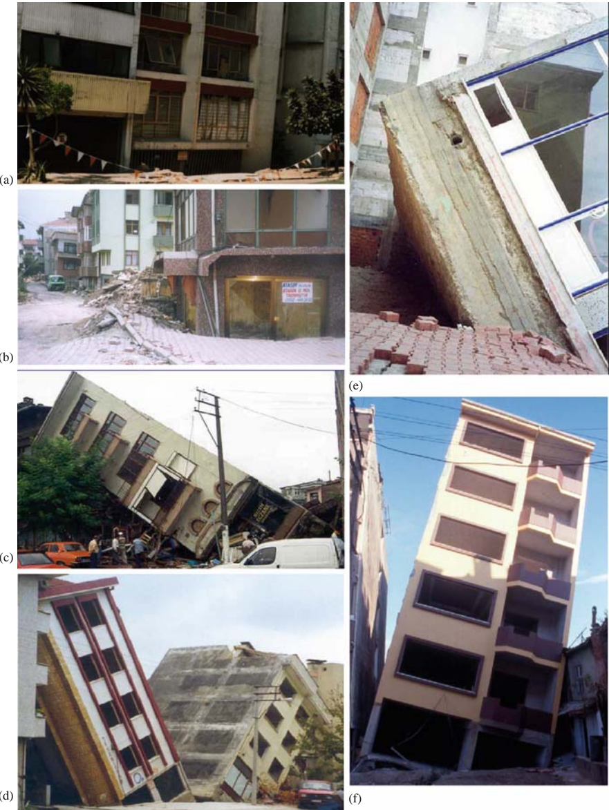
Fig. 2.18 Bearing capacity failures at: (a) in Mexico City (1985) (b)–(f) Adapazari (TR) in the 1999 Kocaeli earthquake (courtesy G. Gazetas, NTUA). (See also Colour Plate 6 on page 720)
