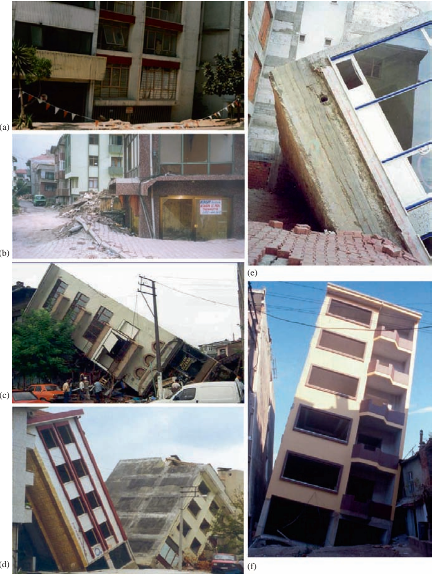
Plate 6 Bearing capacity failures at: (a) in Mexico City (1985) (b)–(f) Adapazari (TR) in the 1999 Kocaeli earthquake (courtesy G. Gazetas, NTUA). (See also Figure 2.18 on page 109)
